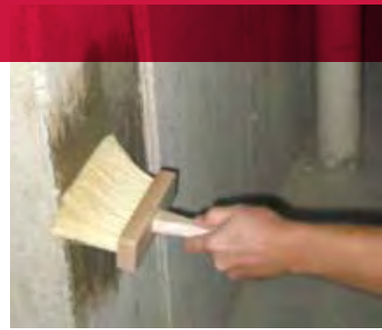
Applying waterproofing material with a masonry brush.
