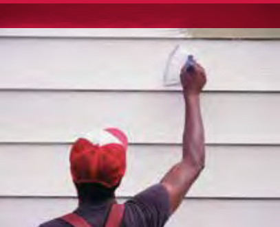
Applying paint to clap board siding.
