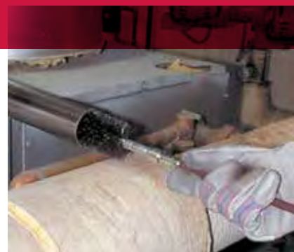
Cleaning boiler pipes with a flue brush.
