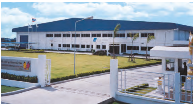
NT TOOL (THAILAND) CO., LTD. (OFFICE/FACTORY)
